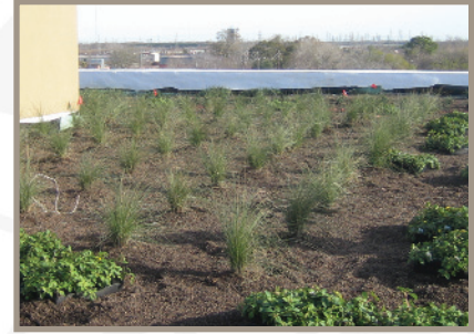
Green roofs provide many benefits — one being a recreation area for occupants.
